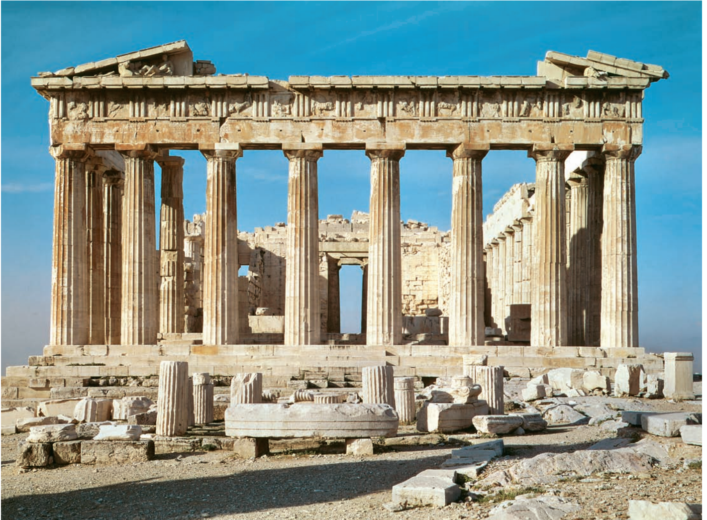
7.17 East end of the Parthenon, Athens, 447–438 B.C. Pentelic marble, 111 × 237 ft. (33.8 × 72.2 m). Once through the Propylaea at the western edge of the Acropolis, the visitor emerges, facing east. Ahead and a little to the right are the remains of the western façade of the Parthenon. Its damaged state reflects centuries of neglect and misuse. In the 5th century A.D. the Parthenon became a Christian church, and in the 15th century the Turks conquered Athens and converted the temple into a mosque. They stored gunpowder in the building! When it was shelled by artillery in 1687, most of the interior and many sculptures were destroyed. Centuries of vandalism and looting, plus modern air pollution, have further contributed to the deterioration of the Parthenon.
