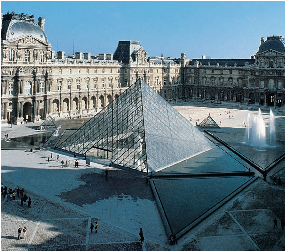
31.11 I. M. Pei, Louvre Pyramid, Paris, 1988. The pyramid is 65 ft. (19.80 m) high at its apex and 108 ft. (32.90 m) wide; it contains 105 tons (107,000 kg) of glass.
