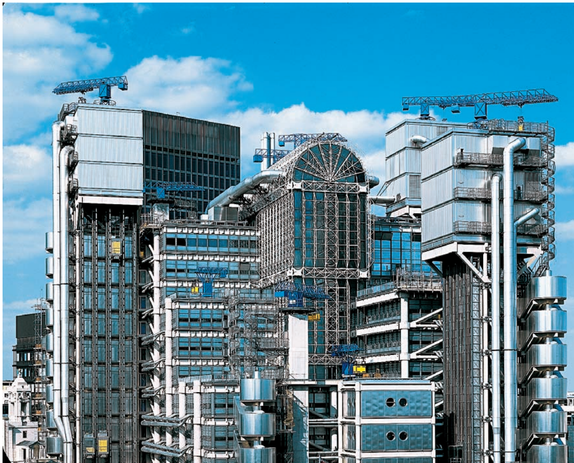
31.12 Richard Rogers, Lloyd's Building, London, 1986. Rogers wrote that “esthetically one can do what one likes with technology . . . but we ignore it at our peril. To our practice, its natural functionalism has an intrinsic beauty.” In the Lloyd's Building, Rogers has fulfilled his philosophical view of uniting technology with aesthetic appeal.
