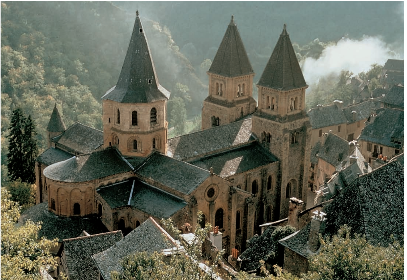
12.1 Aerial view of Sainte-Foy, Conques, Auvergne, France, c. 1050–1120. Apart from two 19th-century towers on the west façade, Sainte-Foy stands today as it did in the 12th century. It has a relatively short nave, side aisles built to the full height of the nave (so that there is no clerestory lighting), and a transept. The belfry , or bell tower, rises above the roof of the crossing .
