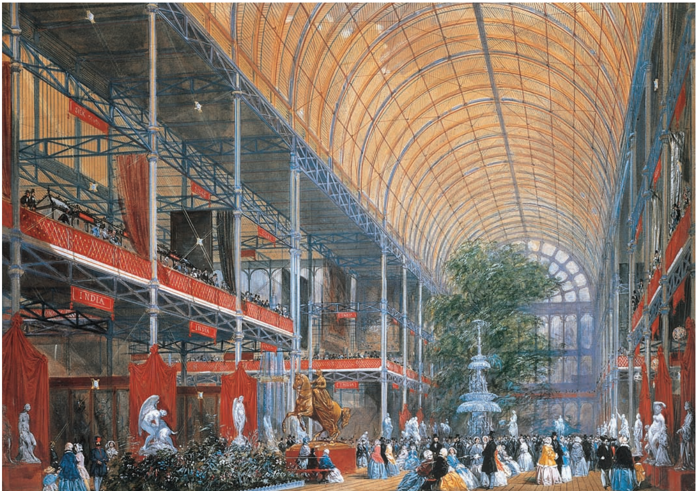
23.19 Joseph Paxton, Crystal Palace, London, 1850–51. Cast iron, wrought iron, and glass. Engraving (R. P. Cuff after W. B. Brongner). Victoria and Albert Museum, London, England. The Crystal Palace was 1,850 feet (564 m) long (perhaps an architect’s pun on the year in which it was built) and 400 feet (122 m) wide. It covered an area of 18 acres (7.3 ha), enclosed 33 million cubic feet (934,000 m 3 ) of space (the largest enclosed space up to that time), and contained more than ten thousand exhibits of technology and handicrafts from all over the world.
