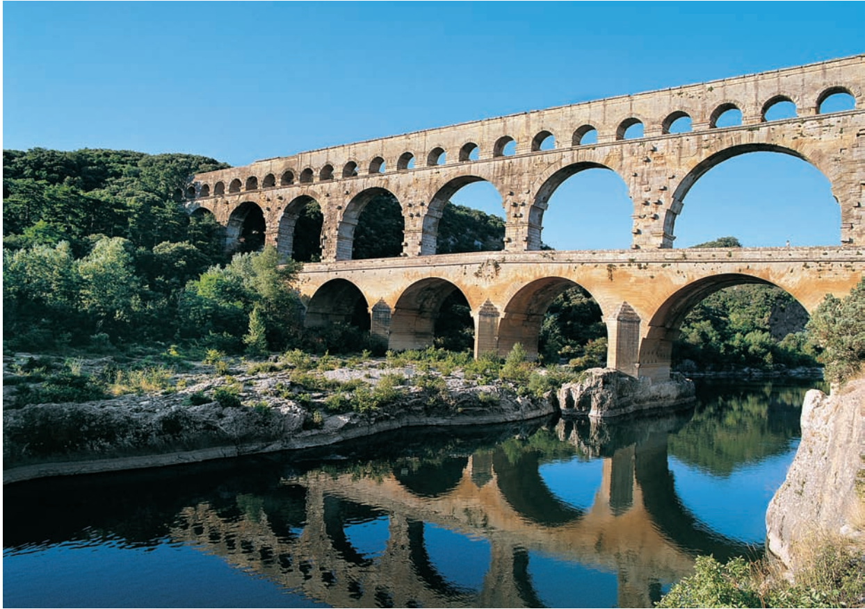
9.14 Pont du Gard, near Nîmes, France, late 1st century B.C. Stone, 854 ft. (260 m) long, 162 ft. (49 m) high. The aqueduct system maintains a constant decline of 1 in 3,000, resulting in a total drop of only 54 feet (16.5 m) over its whole length of 30 miles (48 km).
