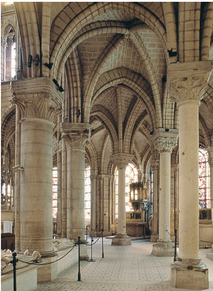
13.2 Interior of Saint-Denis. Each chapel bay has a pair of large stained-glass windows, delicate columns, and rib vaults. The ambulatory and chapels have merged to form a series of spaces illuminated by large windows supported by a masonry frame. Suger described the new effect as “a circular string of chapels, by virtue of which the whole [sanctuary] would shine with the miraculous and uninterrupted light of the most luminous windows.”
