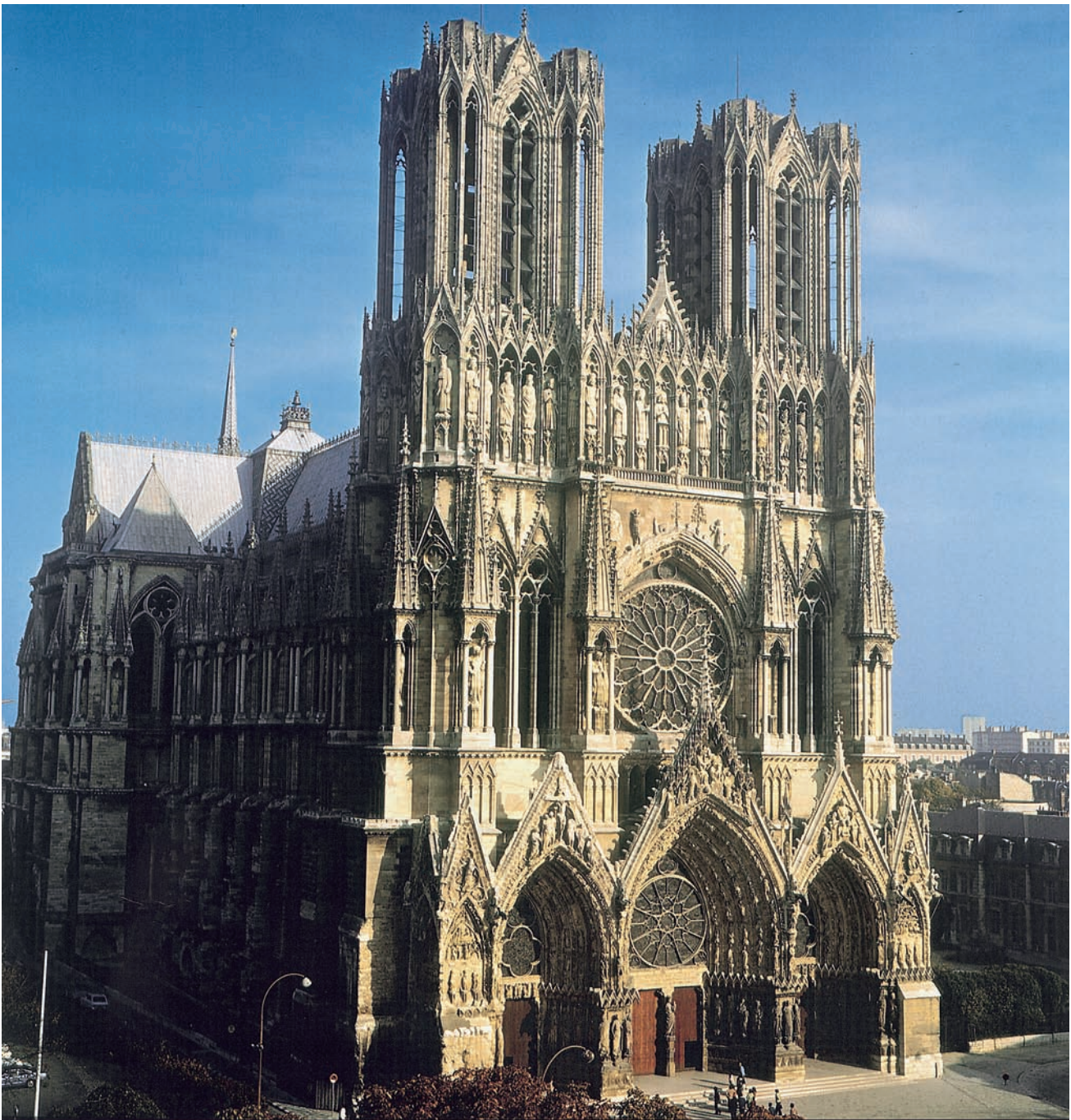
13.20 West façade, Reims Cathedral, France, begun 1211. The window space has been dramatically increased at Reims as a result of continual improvements in the buttressing system. The tympanums on the façade, for example, are filled with glass rather than stone. At Reims the portals are no longer recessed into the façade but are built outward from it.
