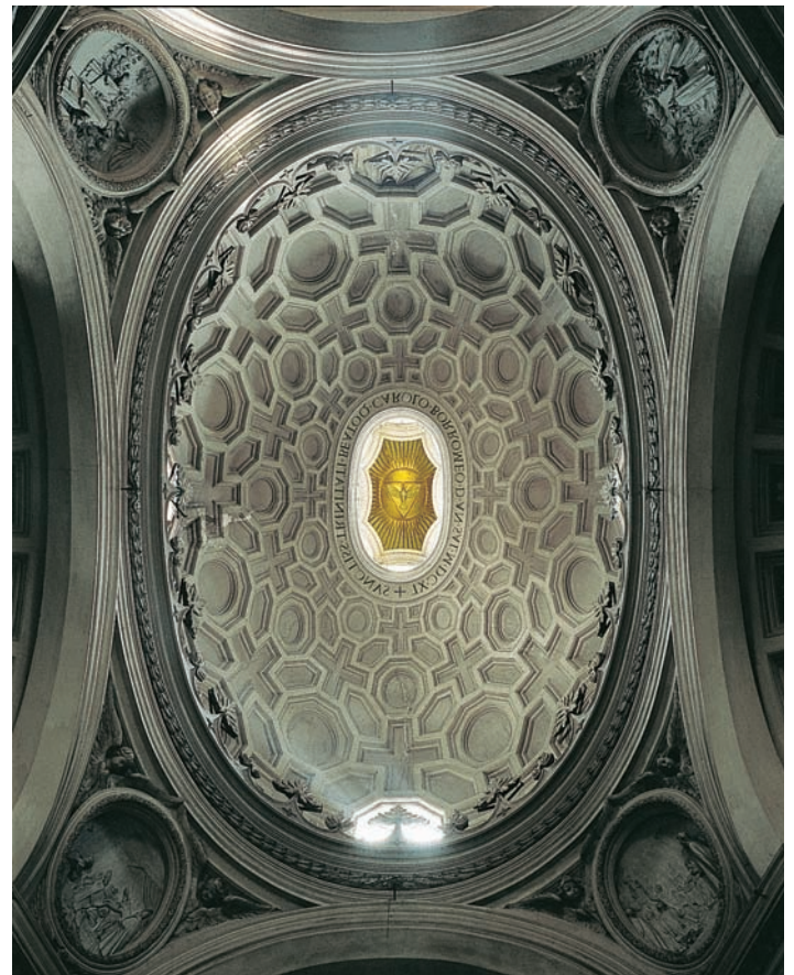
19.7 Francesco Borromini, interior dome of San Carlo alle Quattro Fontane, Rome. The dome is illuminated on the interior by windows at its base and contains coffers in the shape of hexagons, octagons, and crosses. At the center of the dome, an oval oculus contains a triangle: a geometric symbol of the Trinity and an emblem of the Trinitarian Order that commissioned the church.
