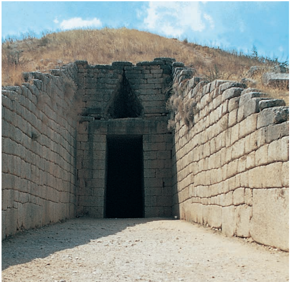
6.16 Façade and dromos of the “Treasury of Atreus,” Mycenae, 13th century B.C. Originally the door was framed by half-columns made of gypsum.
