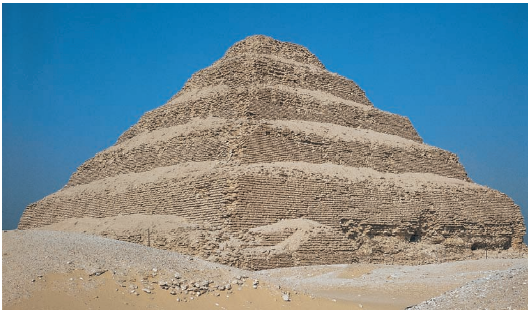
5.4 Step pyramid, funerary complex of King Zoser, Saqqara, Egypt, 2630–2611 B.C. Limestone, 200 ft. (61 m) high. Its architect, Imhotep, was a priest at Heliopolis and is reputed to have been the first Egyptian to build monumental stone structures. His name is inscribed inside the pyramid, where he is designated "First after the King of Upper and Lower Egypt." He became a legendary figure in ancient Egypt, revered for his wisdom as a magician, astronomer, and healer, and was worshiped as a god.
