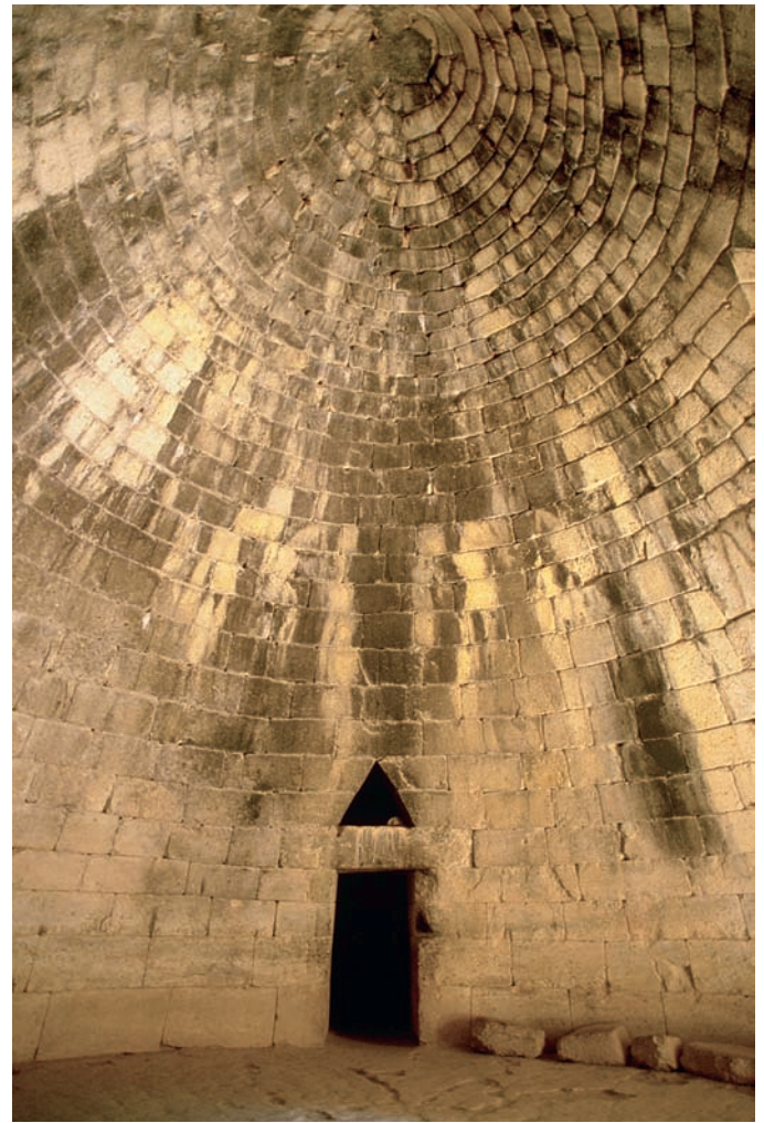
6.18 (Above) Interior of a tholos tomb, showing the entrance lintel and a door to the side chamber. "Treasury of Atreus," Mycenae, 13th century B.C. Diameter of interior 43 ft. (13 m), height 40 ft. (12 m); doorway 17 ft. 8 in. × 8 ft. 10 in. (5.4 × 2.7 m).
